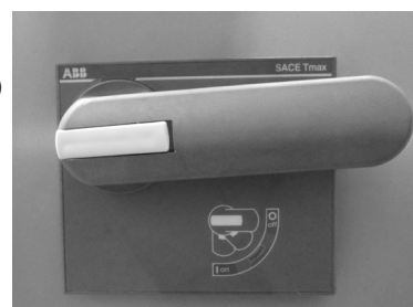
Figure 3 Main Breaker (Shown in the OFF position.)
