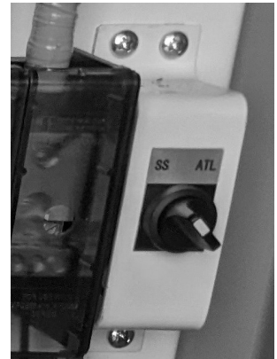
Figure 2 SS/ATL Switch (Inside Control Panel.)
