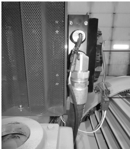
Figure 13 Disconnect fan from fan controller
