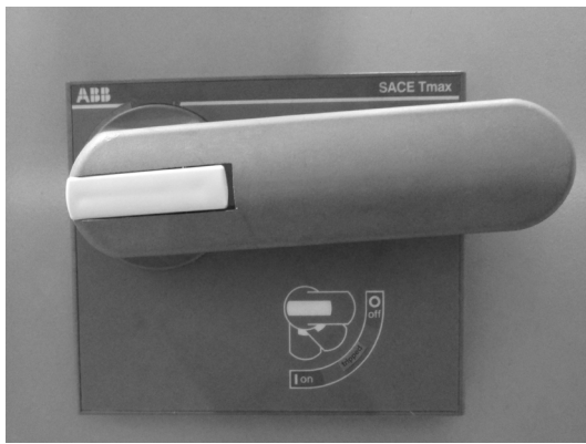
Figure 3 Main Breaker (Shown in the OFF position.)
