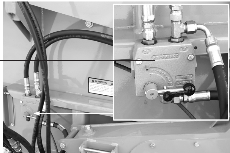
flow control valve with valve in the full open position
